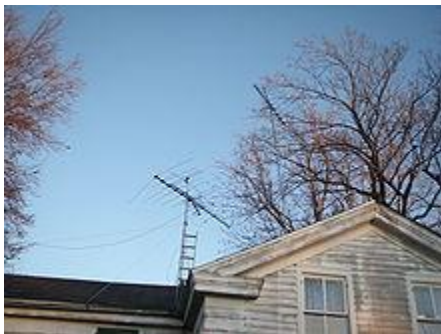
Two aerials setup on a roof. Spaced horizontally and vertically
